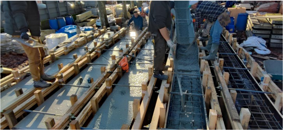
Ongoing casting of the RC beams for the competition
